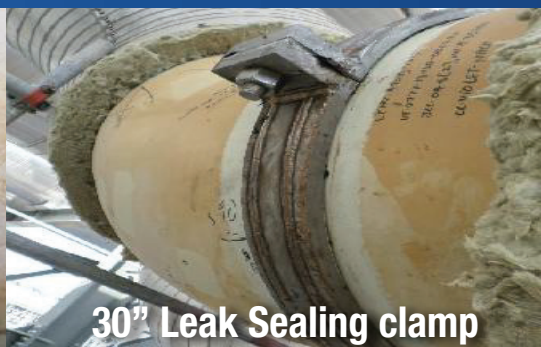
5 mm pin hole on 30" SS line
