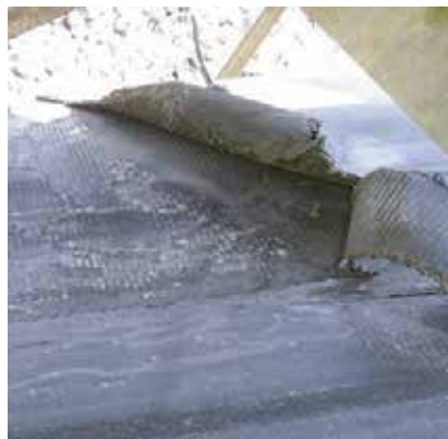
Before Repair: Large tear in belt due to rocks getting caught under the scraper blade.
