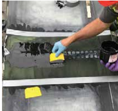
Before Metal Clips Splice Repair
