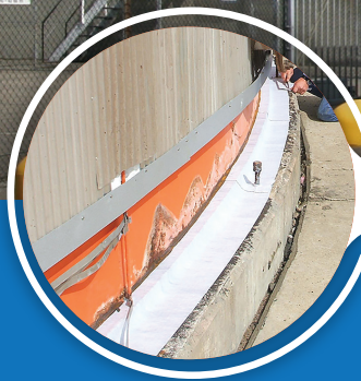
TANK CHIME SEALING
