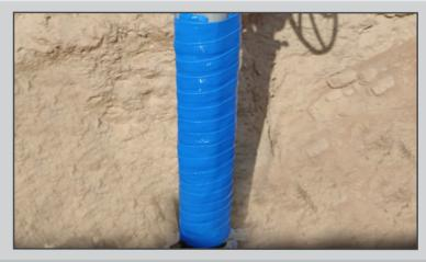
Outer Wrap should be wrapped with tension and a minimum of 50 % overlap. First wrap and termination wrap should be a straight circumference wrap
